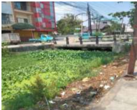
Image 4. A.Yani Road Bridge at KM 4 (Personal Documentation, 2023)
