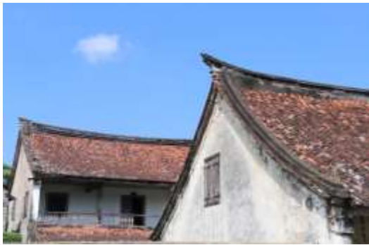
Figure 6. The roof of the Lasem Chinatown Han House. (Source: Personal Documentation, 2024).
