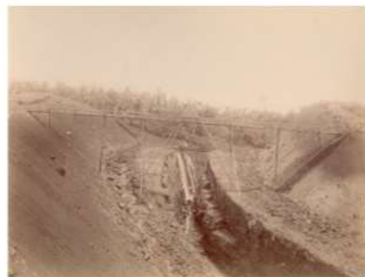
Figure 2: Railway Line Construction Process in West Java Source: KITLV 100069 and KITLV 100069
