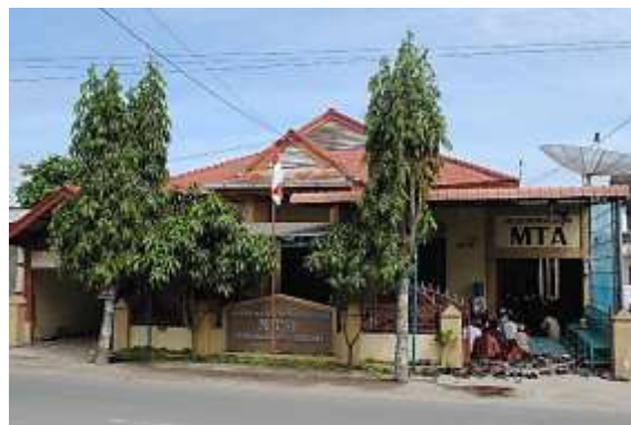
Figure 1. Condition of the MTA Foundation Representative of Deli Medium Before Renovation
