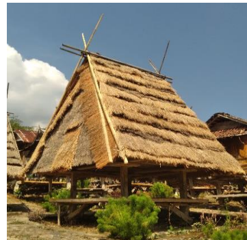
Figure 2. Depicting the structure of a traditional Uma Lengge house
